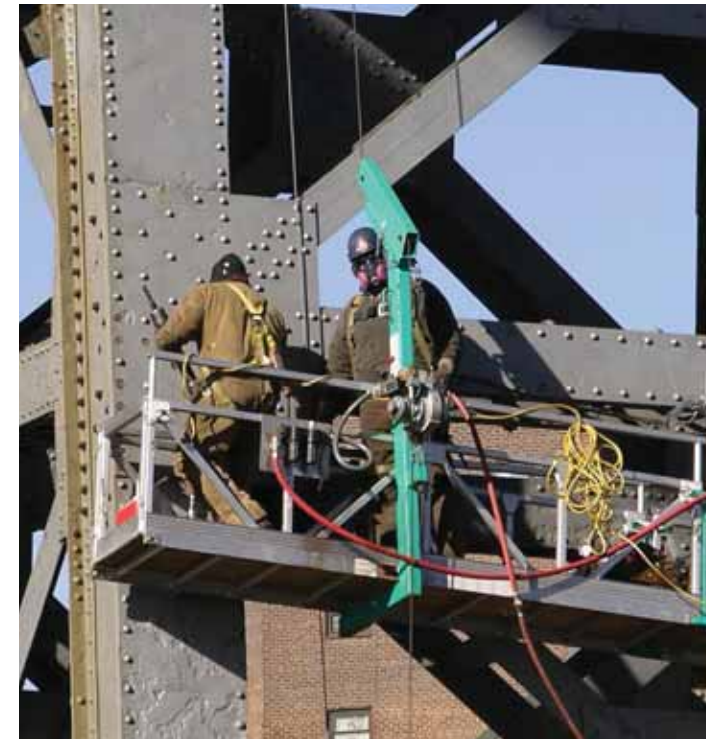
© NYC DOT DIVISION OF BRIDGES
