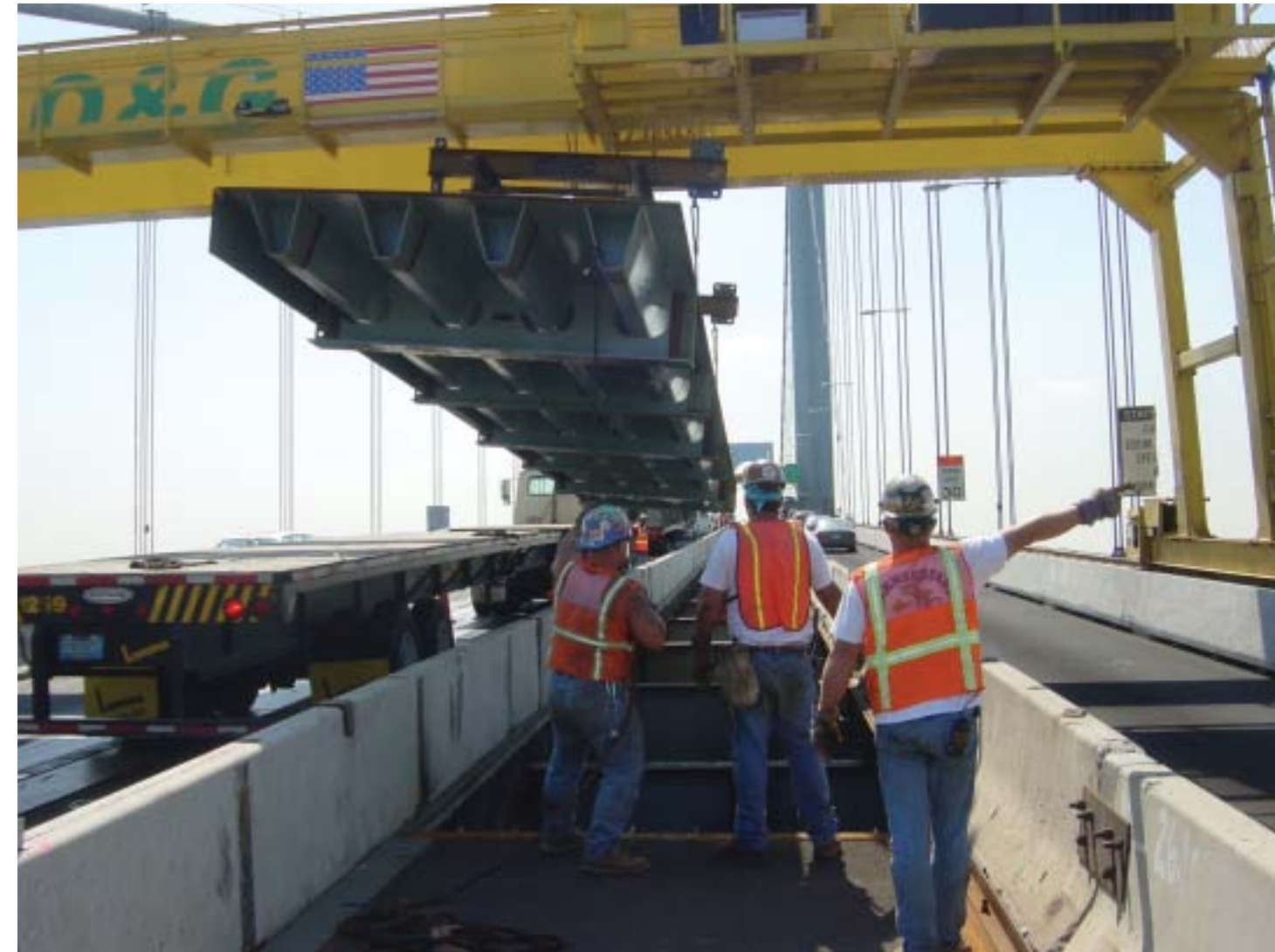
ABOVE A gantry crane lifts a new deck panel into place.
