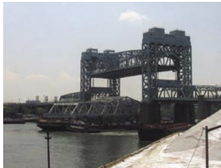
LEFT The new bridge is barged in along the Harlem River.
