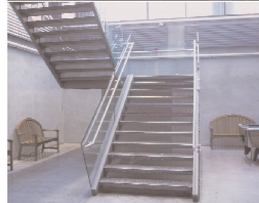
An elegant ornamental metal and terrazzo stair connects the lobby to the lower level...
