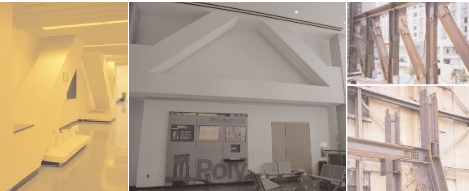
Over the gymnasium, four steel trusses provide an 85-foot clear span for the space while supporting a 4,200-sq.ft.elevated courtyard.
