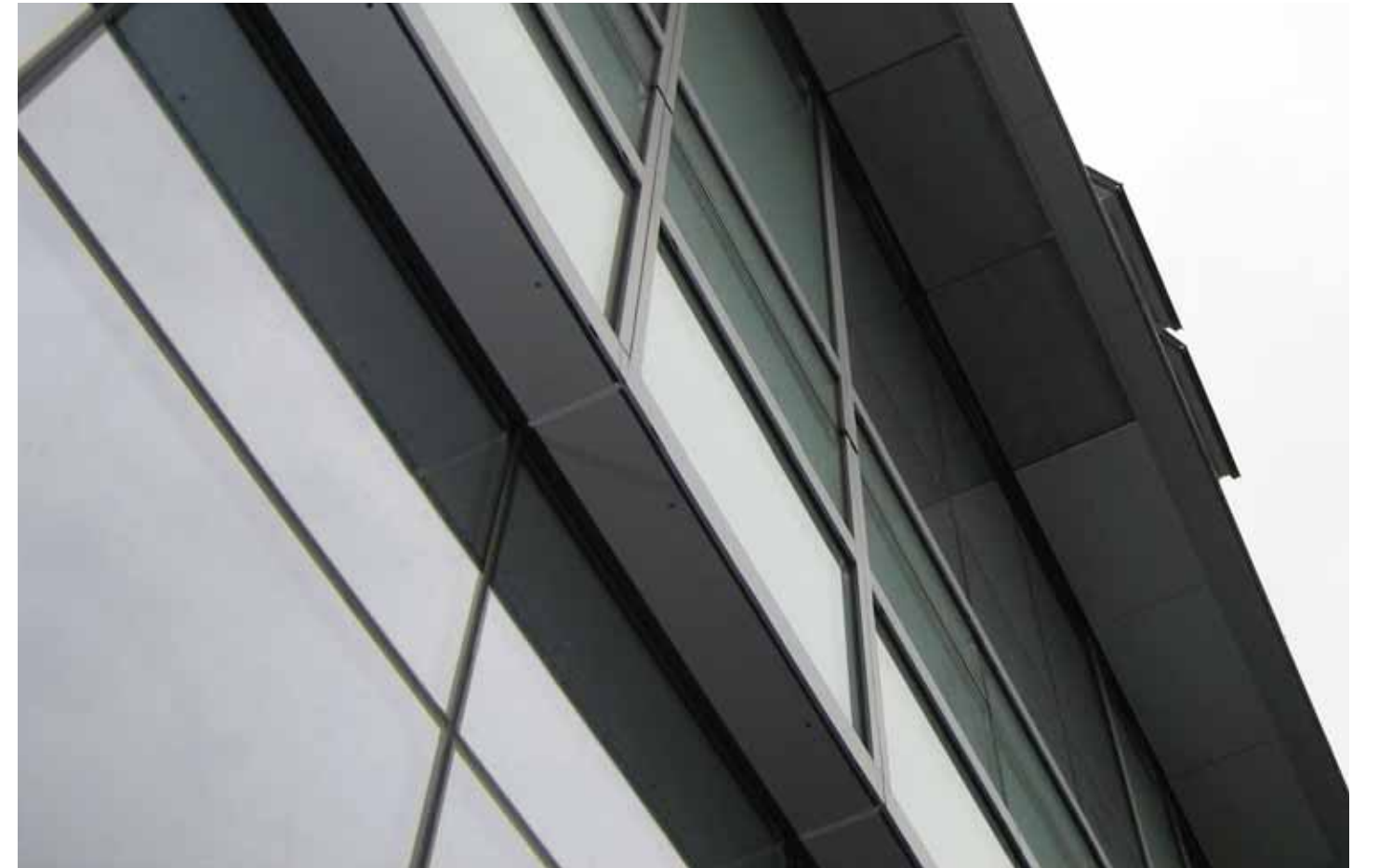
ABOVE The system's sliding and fixed anchors allow for construction tolerances, resulting in an unblemished finish.
