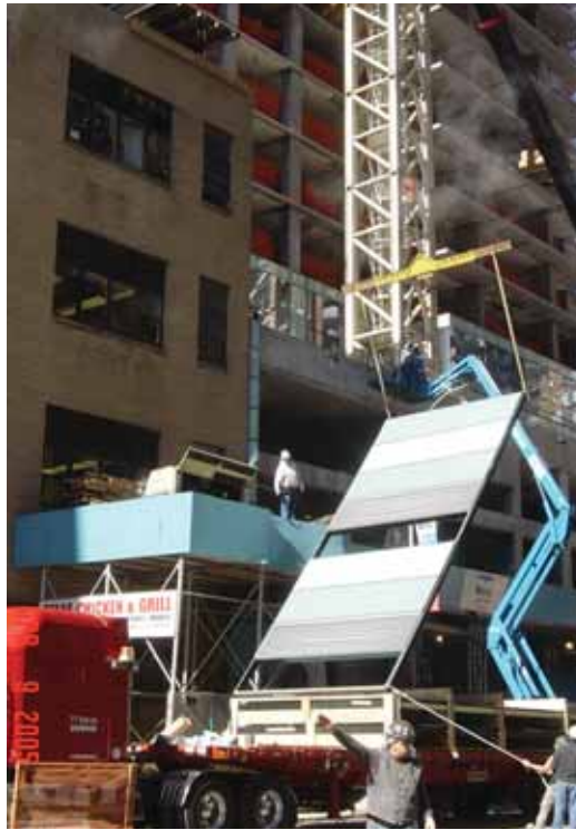
ABOVE As with normal curtain wall, the hybrid system comes in prefabricated panels.
