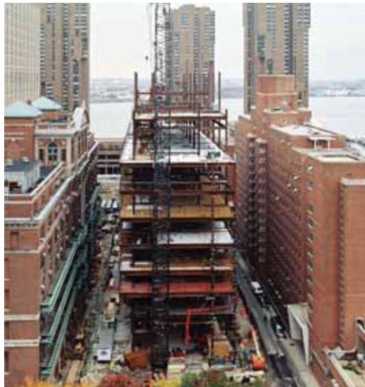
BOTTOM LEFT A tower crane placed alongside the building erected the majority of the structural steel.
