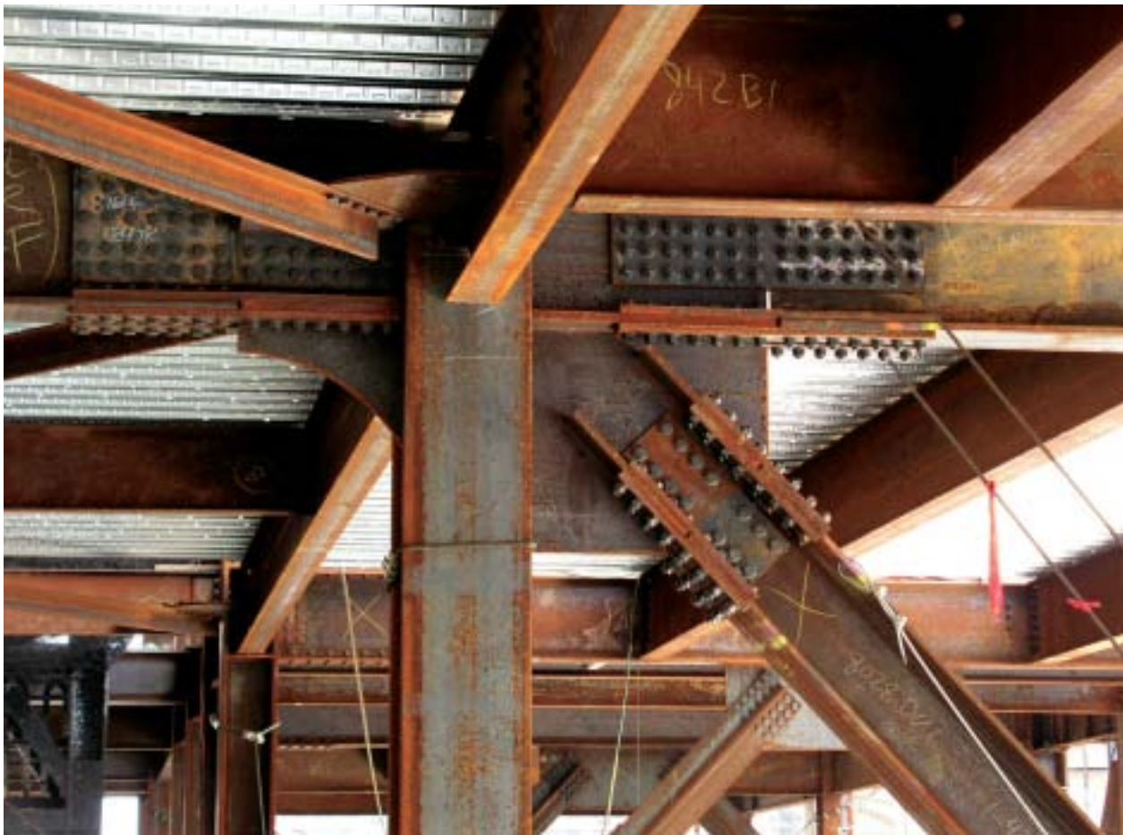
TOP Ironworkers maneuver the mega braces into place.
