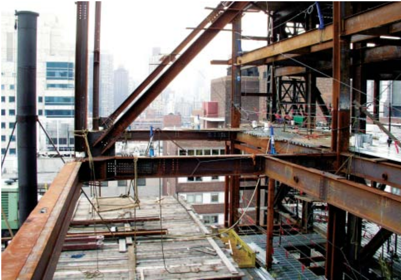
TOP Steel members on the metal decking await erection.
