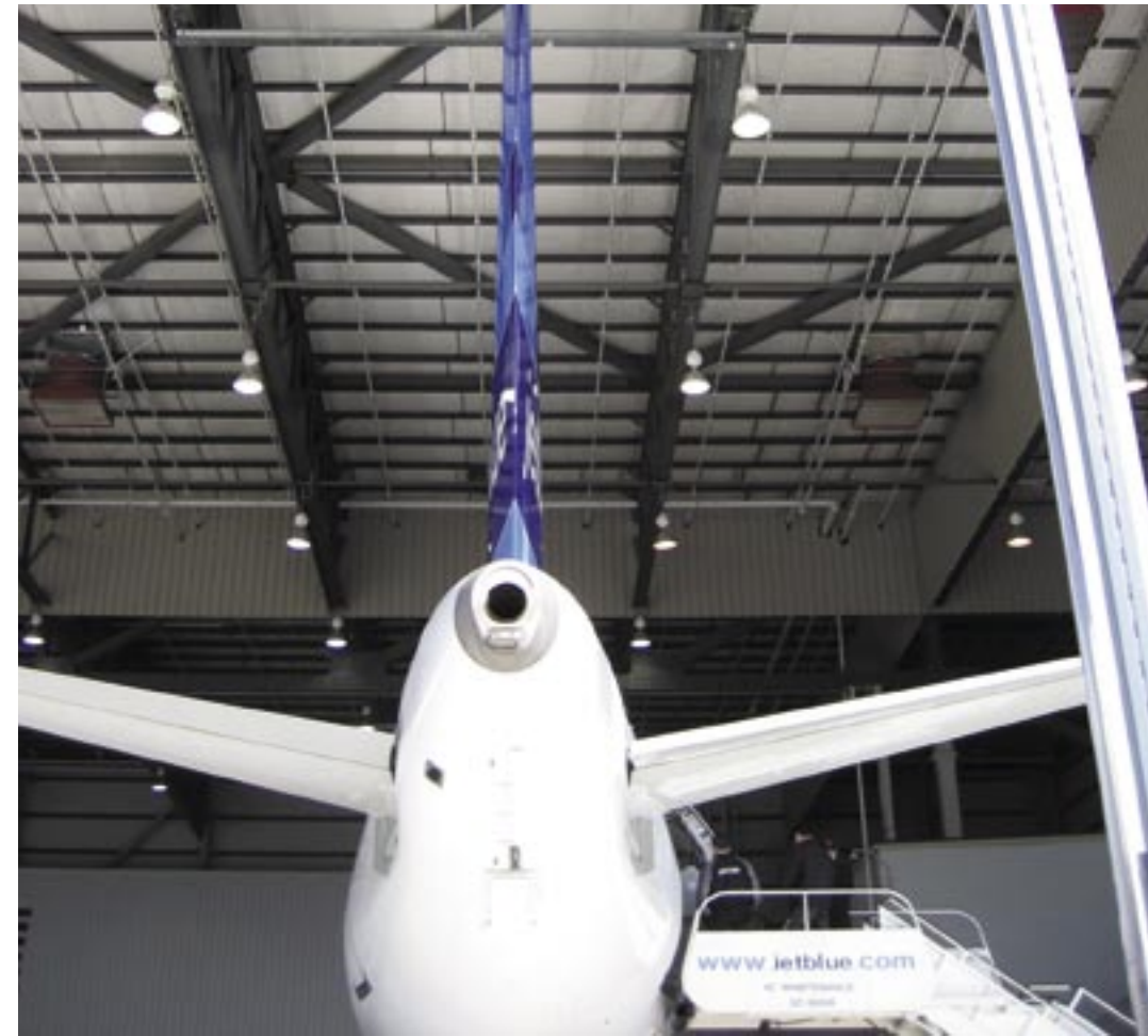
ALL The unique truss system allowed for maximum spans with a relatively shallow truss.
