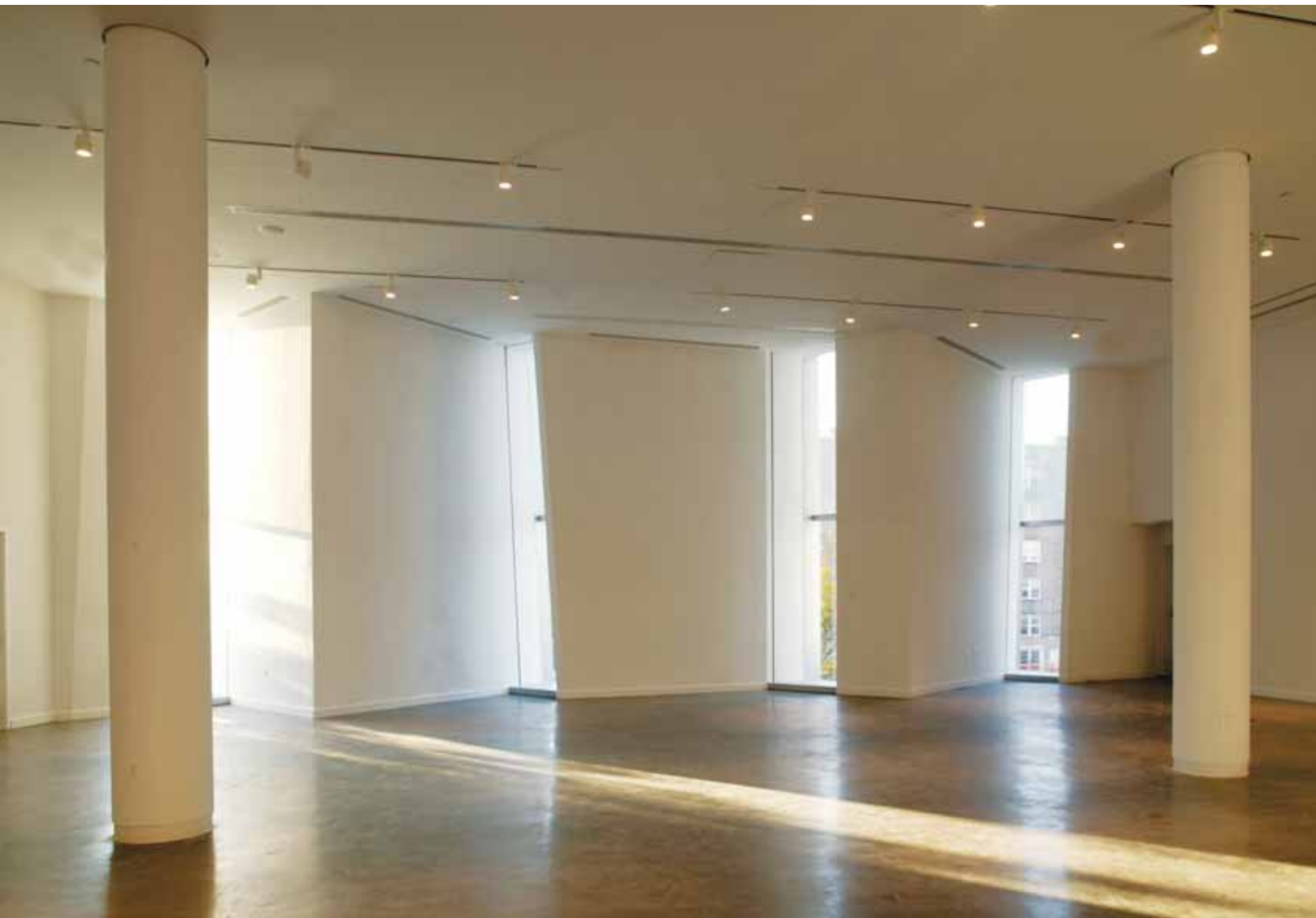
ABOVE AND OPPOSITE The stiffened steel moment frame provides 22 and 20-foot floor to ceiling heights on the first and second stories.
