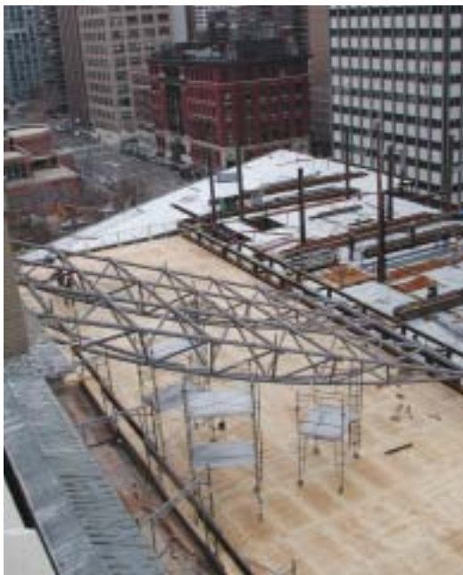
ABOVE The skylight's bow trusses bolt to the addition. Hangars tying back to the existing steel frame connect it to the historic building, while allowing for independent lateral movement in case of seismic activity.
