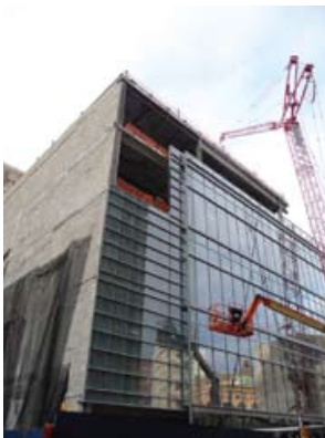
Below, left Steel framing allowed the 50-foot spans necessary for Socratic-style classrooms and auditoriums. Below, center The curtain wall appears to float above the school's first floor. Below, right On the fifth floor, the curtain wall wraps around to form one side of an outdoor terrace.
