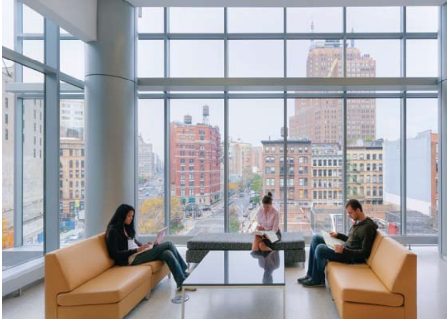
Above Students sit in a northwest corner lounge area. Most of the curtain wall's horizontal supports occur at floor level, emphasizing the feeling of openness.
